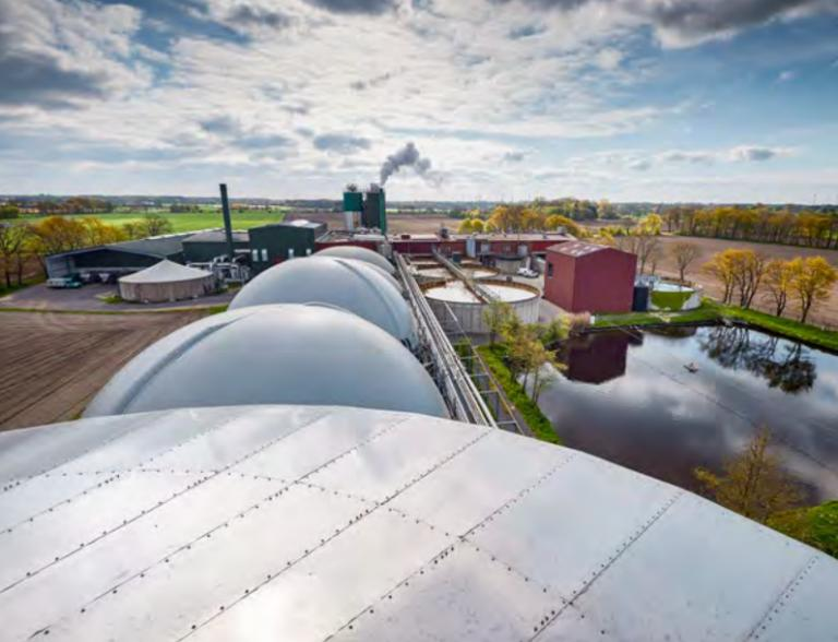
**6** fermenters turn potato remnants into biogas for electricity generation at the Wernsing plant in Addrup.
